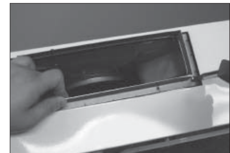
6. Mount starting collar (provided) at rear discharge.
